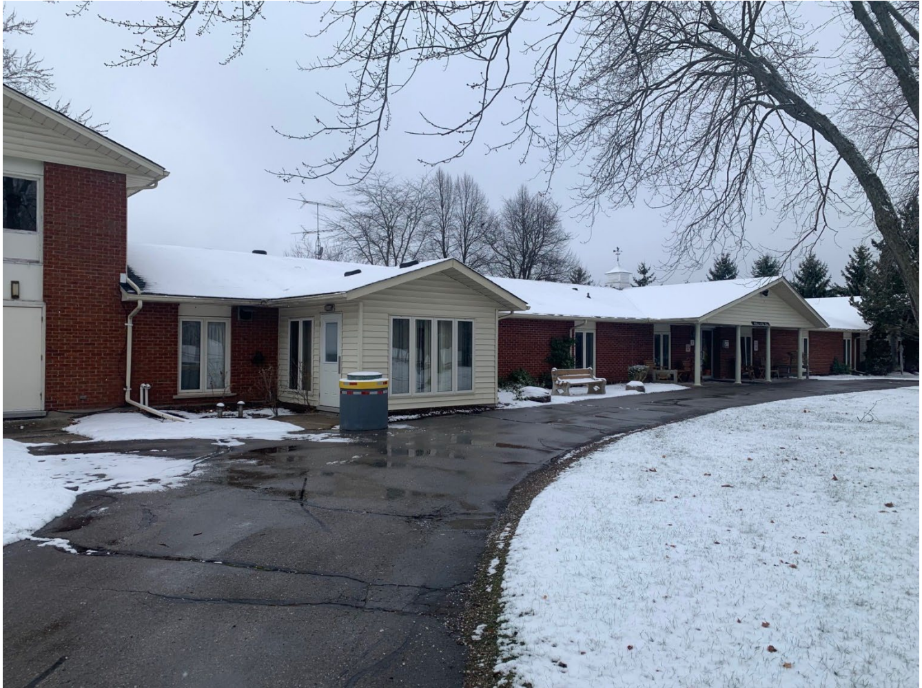
Figure 3- Existing Entrance to Eden House
